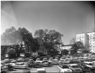
Picture of Smokey Hollow amid Construction of State Buildings
